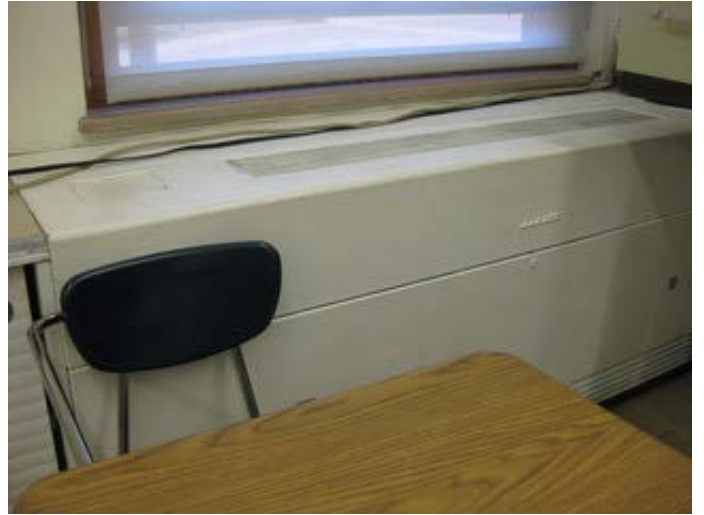
Steam unit ventilator
