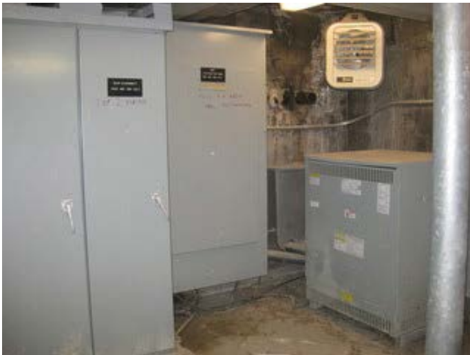
Main Electrical Switch Gear
