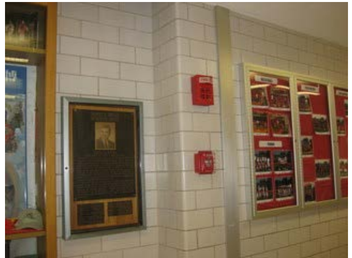
Fire Alarm devices
