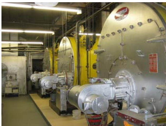
flooding near boilers at floor drains
