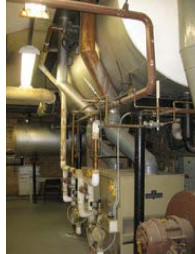
2 Water Heaters and 1 storage tank
