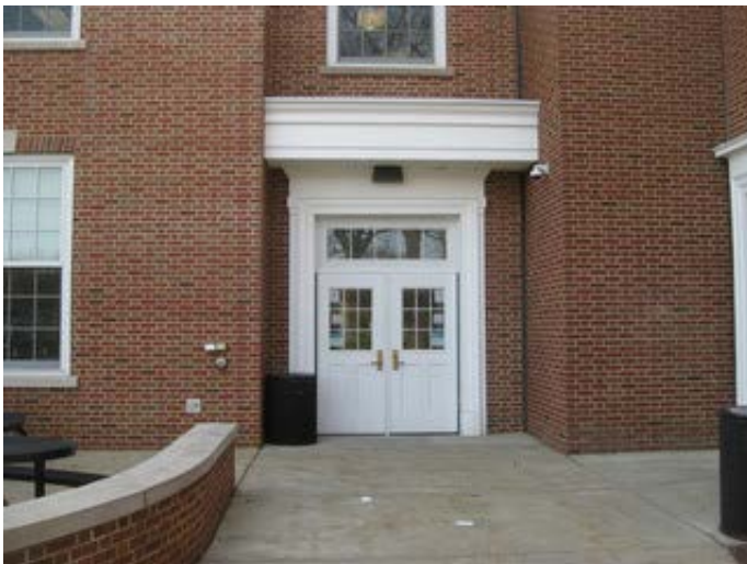
Side entrance door
