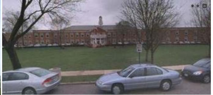
East elevation photo:
