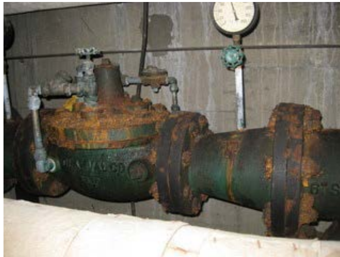
Pressure regulator on 6" water main
