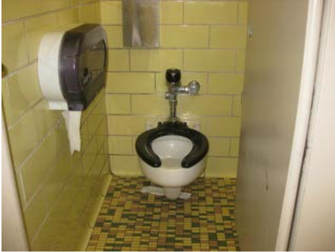
Toilet with sensor faucet
