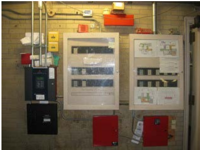
Main Fire Alarm panels
