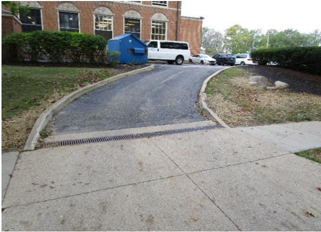
Broken Concrete Curbs
