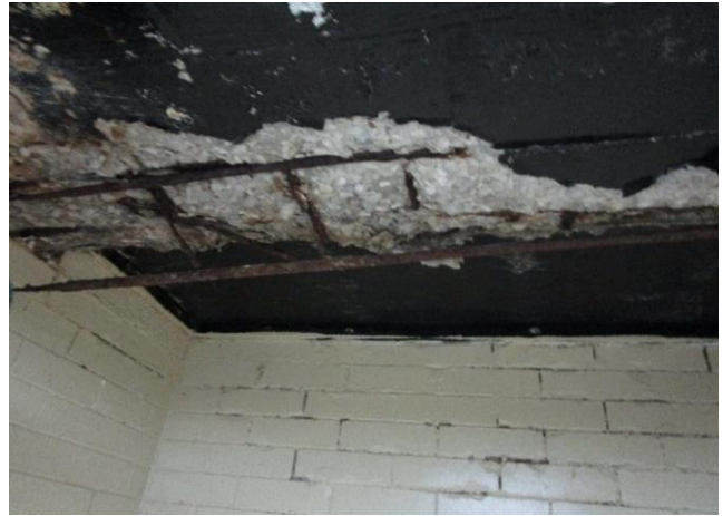
Concrete Deck in Boiler Room Restroom
