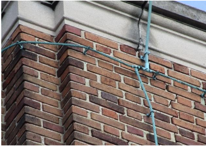
Lightning Strike Damage to Chimney
