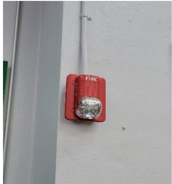
Typical Notification Device
