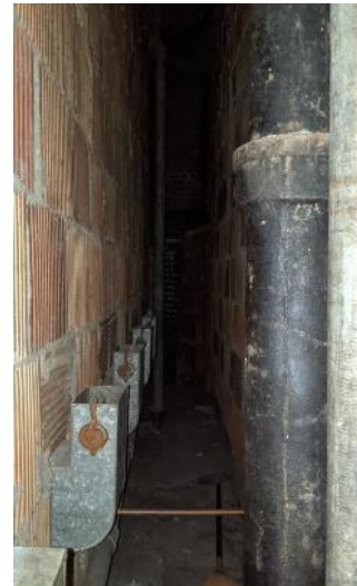
Toilet Exhaust in plumbing chase
