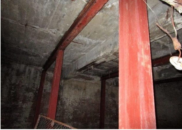
Concrete Deck in Coal Room
