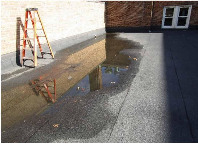
Ponding on Roof
