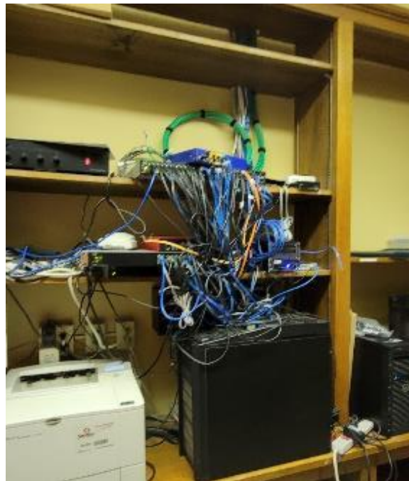
Servers and Patch Panels
