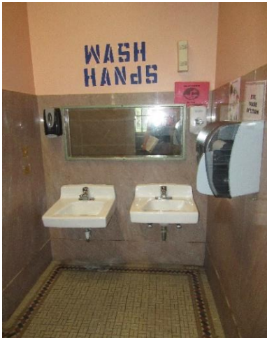
Typical Restroom Lavatory
