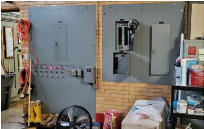
Main Distribution Panels
