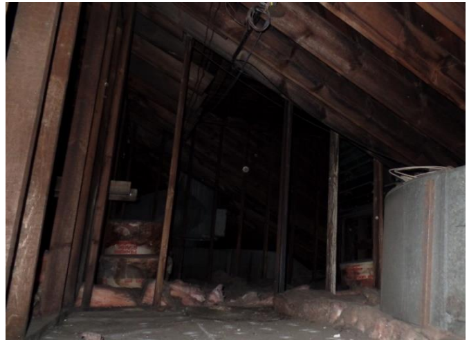
Typical Wood Structure at Sloped Roofs
