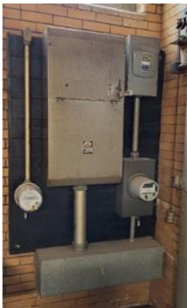
Main Electrical Disconnect
