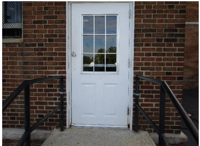
Exterior Door to Gymnasium
