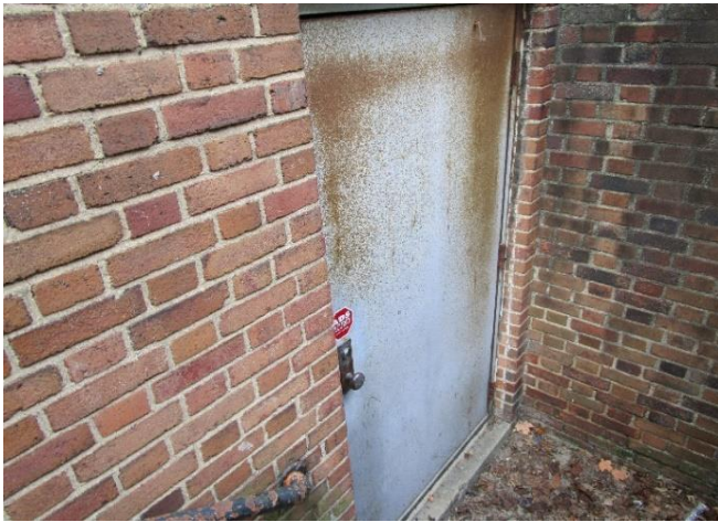
Exterior Door to Boiler Room
