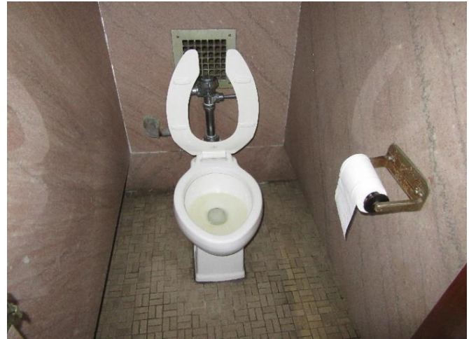
Typical Restroom Stall
