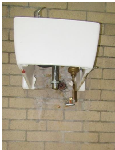
Non-Functional Drinking Fountain
