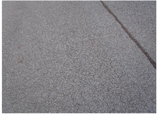
Alligatored Built Up Roofing
