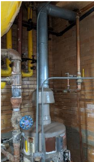
Domestic Hot Water Heater
