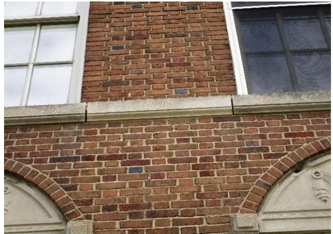
Damaged Stone and Missing Grout
