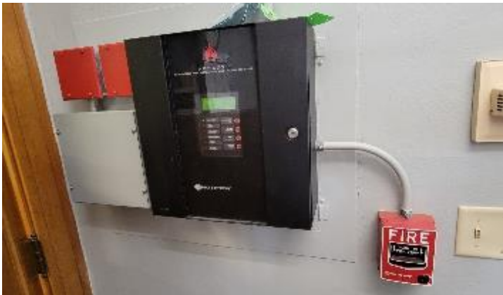
Fire Alarm Control Panel
