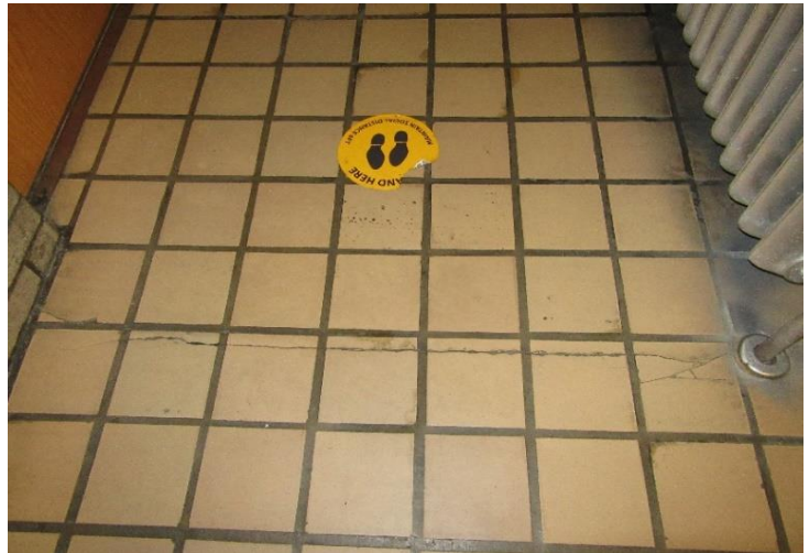
Typical Corridor Flooring
