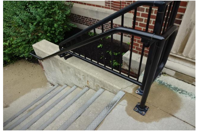
ADA Compliant Handrails
