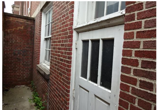
Wood Door to Basement Level
