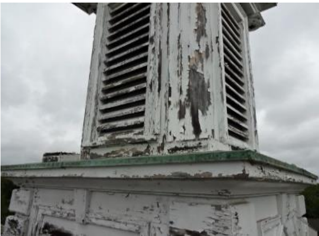
Cupola to be Replaced
