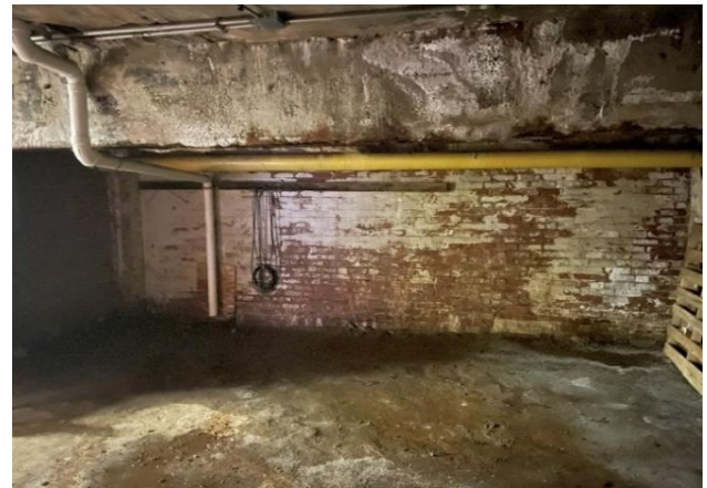
Coal Room Walls
