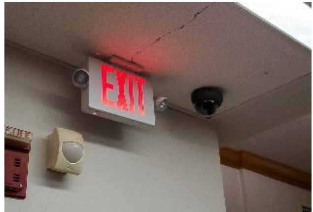
Security Camera and Motion Detector
