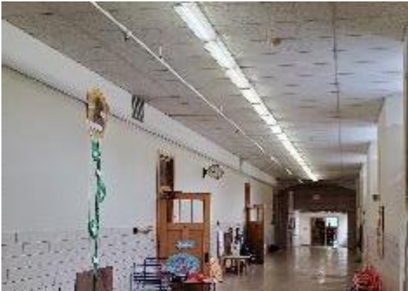
Typical Corridor Lighting
