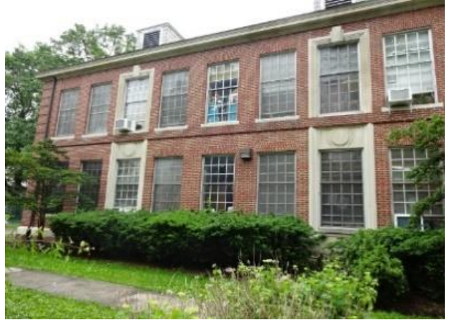
Windows to be Replaced
