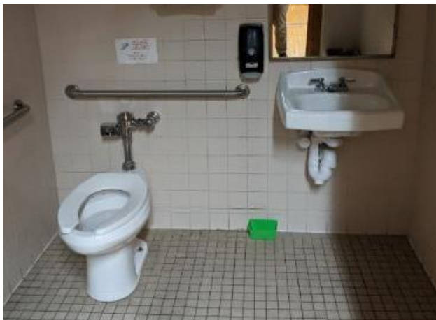
Staff Restroom in 1990 Addition
