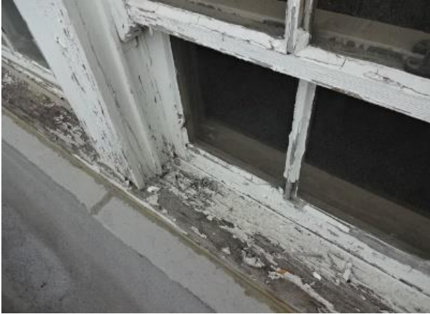
Window to be Replaced
