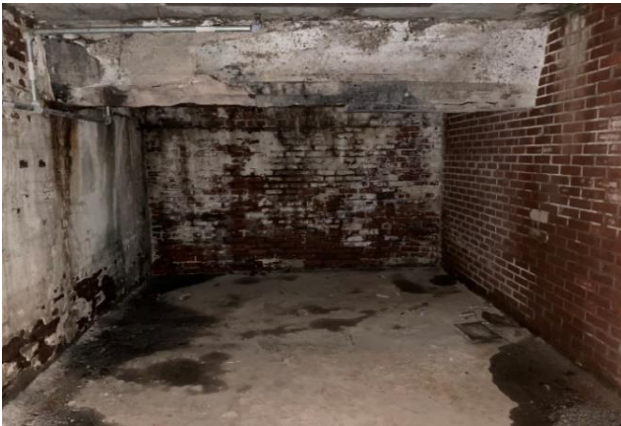
Concrete Beam in Coal Storage Room
