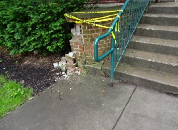
North Steps to be Repaired
