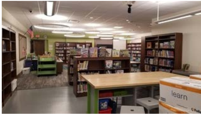
Lighting in media center
