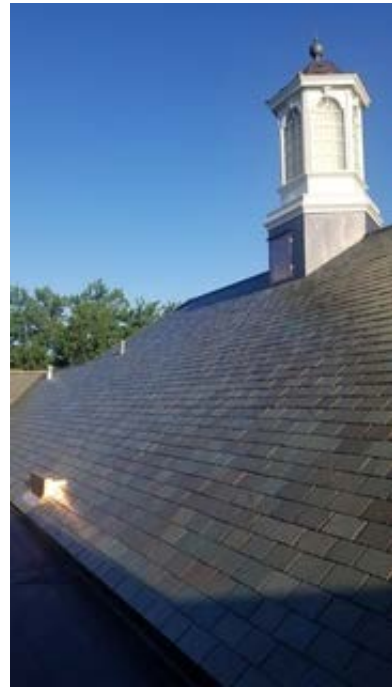
Slate roof at 1927 original construction
