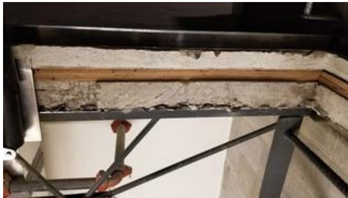
Cast concrete on metal deck at roof structure of 1927 original construction
