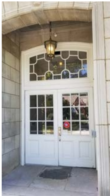
Main entrance doors at 1927 original construction
