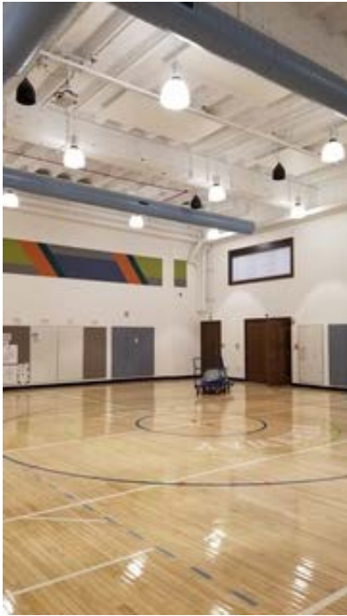
Lighting in gymnasium
