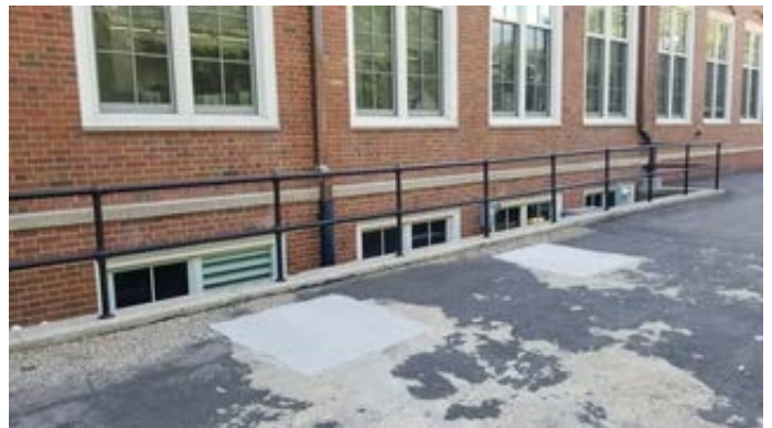
Exterior railings at 1927 original construction
