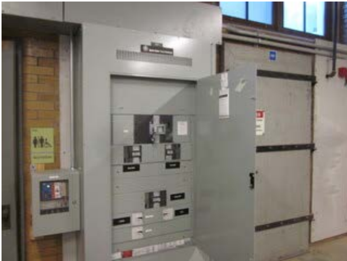
Main distribution panel
