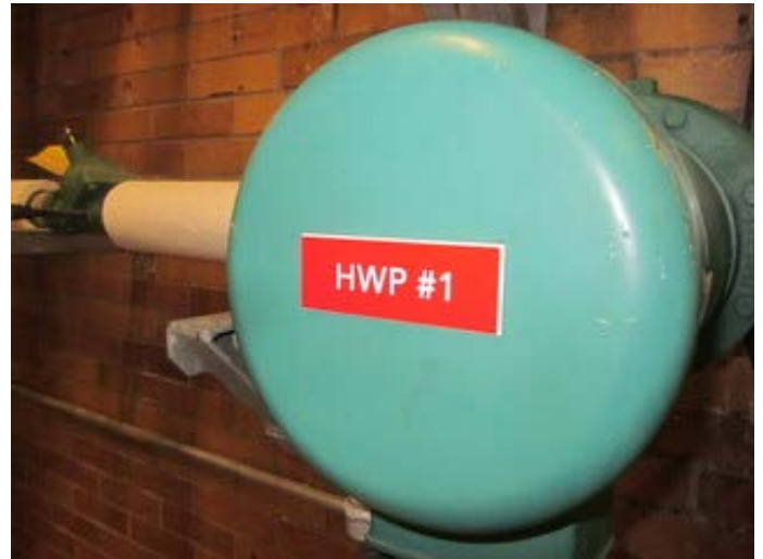
Hot water circulating pump
