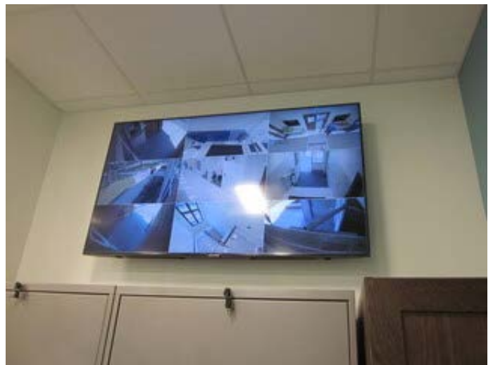
Security camera monitor in main office
