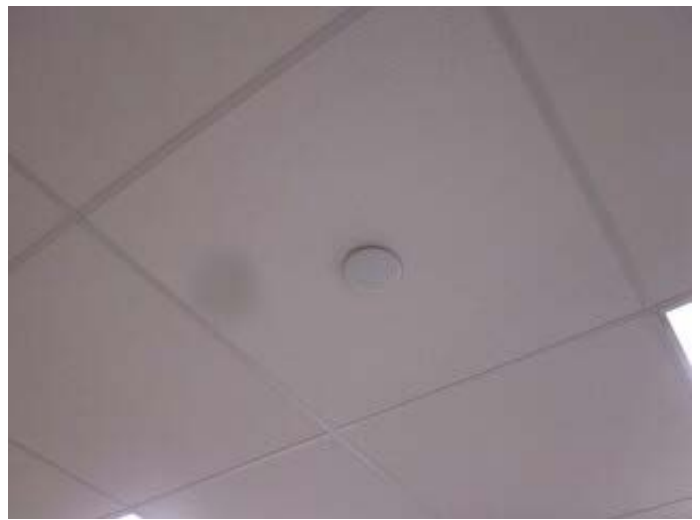
Recessed ceiling mounted sprinkler head
