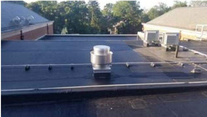
Flat roofs over 1927 original construction and 2020 addition
