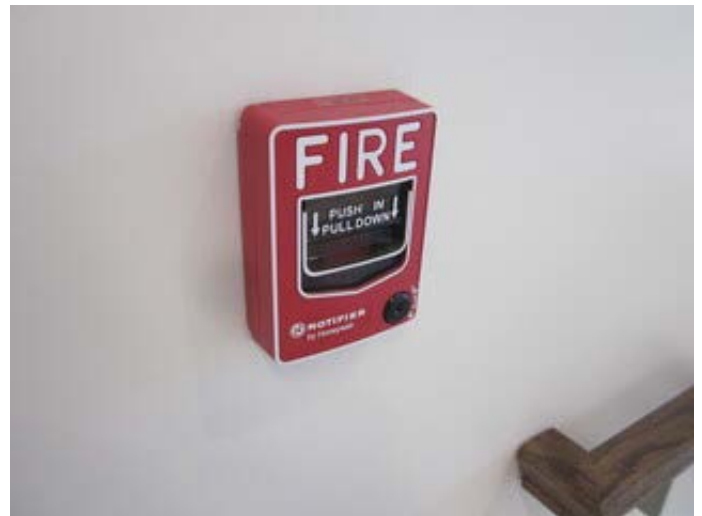
Fire alarm pull station
