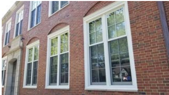
Windows in 1927 original construction
