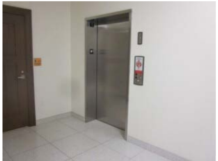
Elevator in 2020 SE and 2nd Floor Media Addition
