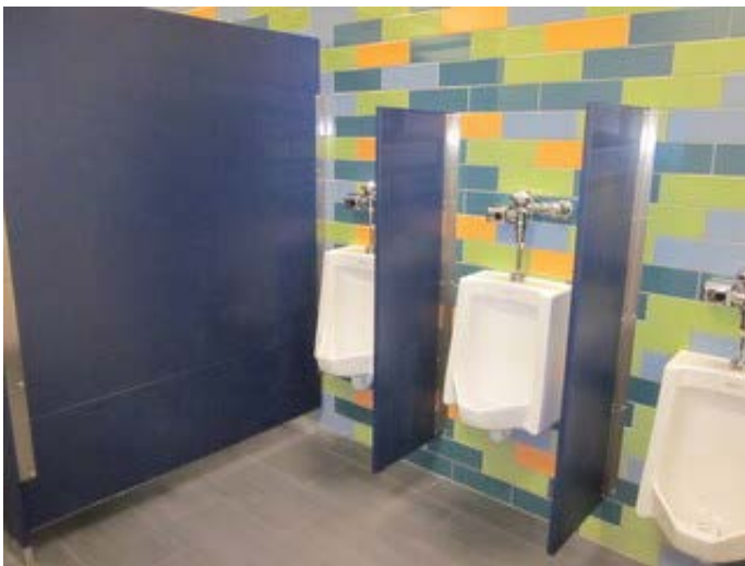
Wall mounted restroom fixtures
