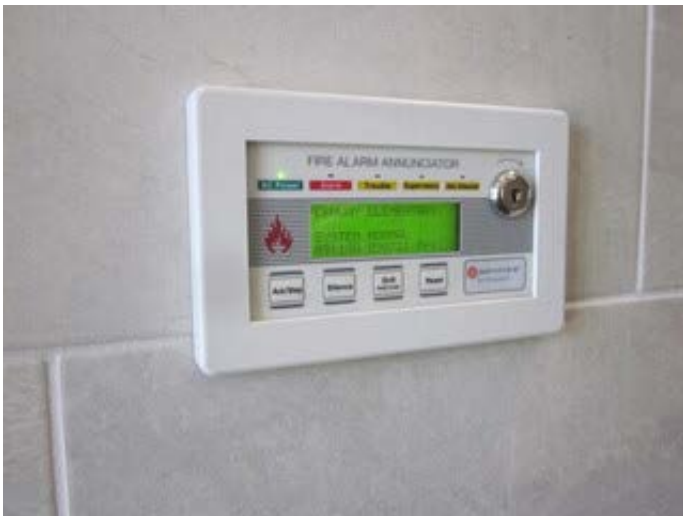
Fire alarm annunciator panel
