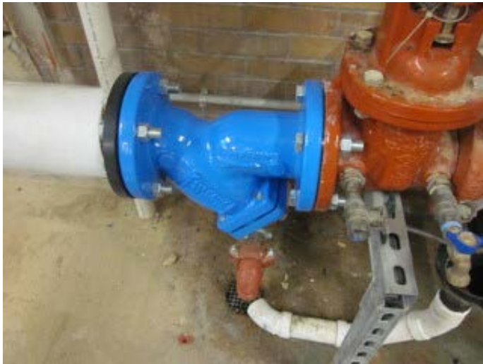
Water service back-flow preventor
