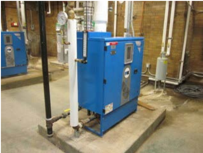
Gas fired boiler
