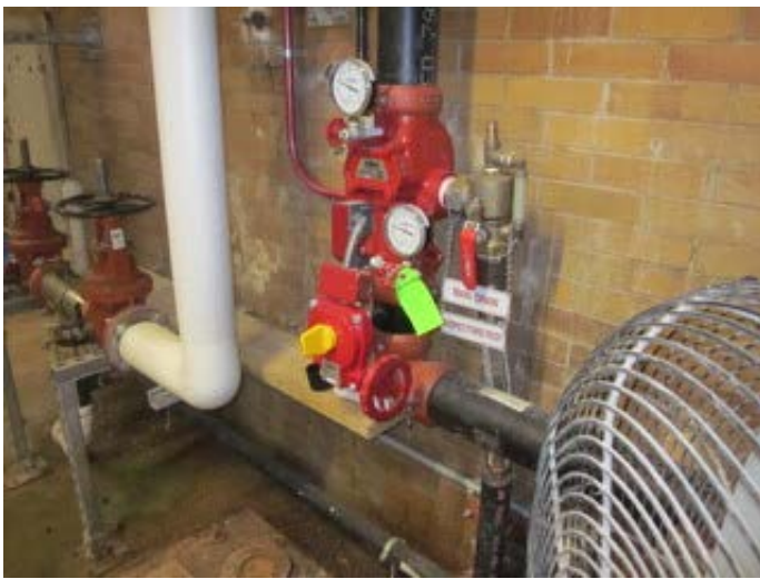
Fire suppression supply piping
