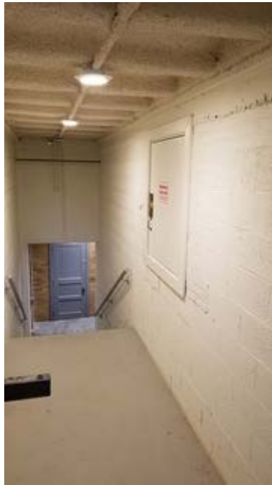
Masonry block foundation walls
