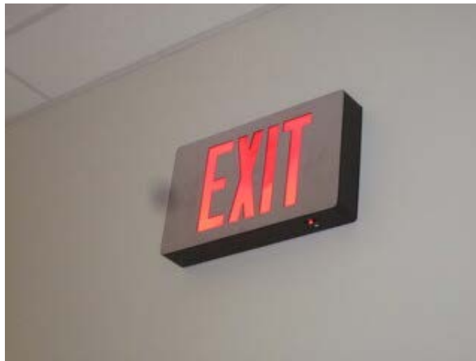
Wall mounted exit signage
