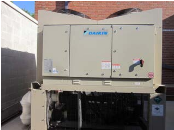
Pad mounted chiller
