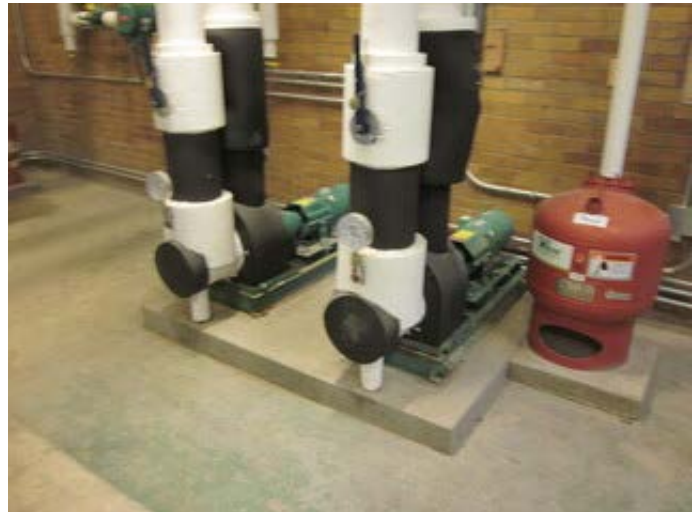
Cold water circulating pumps
