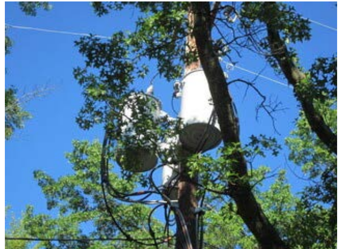
Pole mounted transformers
