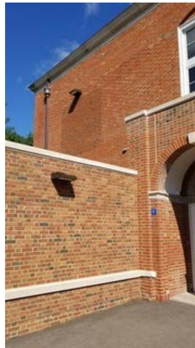
Masonry brick exterior walls
