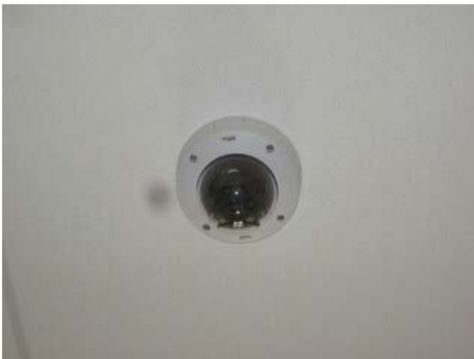
Ceiling mounted security camera
