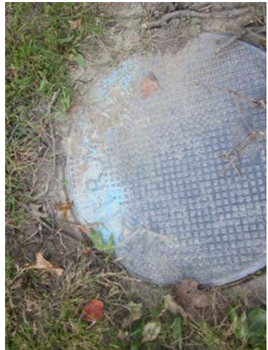
Water service meter pit
