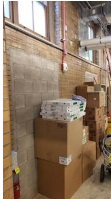
Masonry block and brick foundation walls
