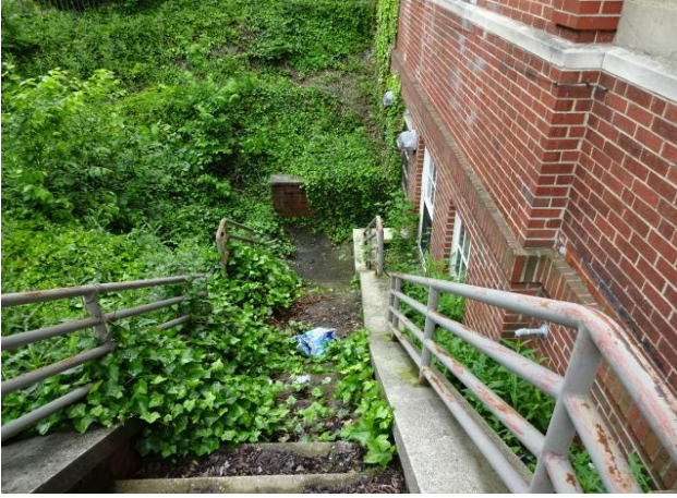
Overgrown Landscaping and Railings
