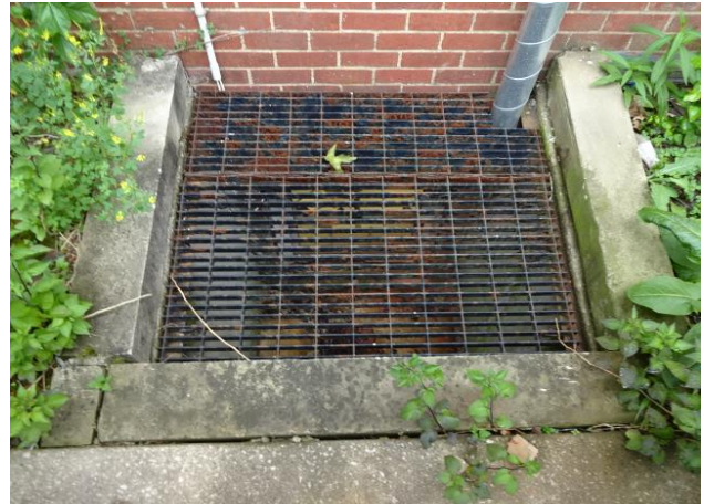
Foundation at Basement Light Well
