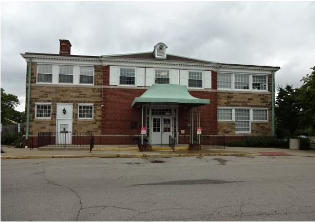
Main Entrance - South Elevation
