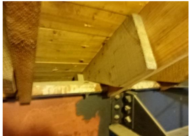
Wood Rafters and Decking
