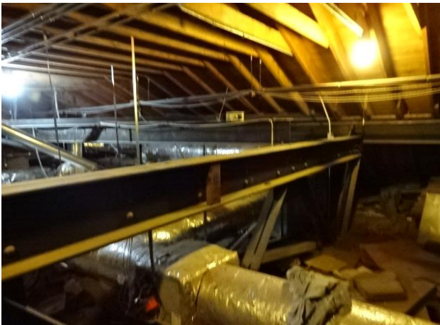
Steel Roof Truss and Wood Rafters
