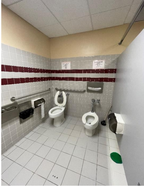
Basement Level Restroom with Extra Fixture
