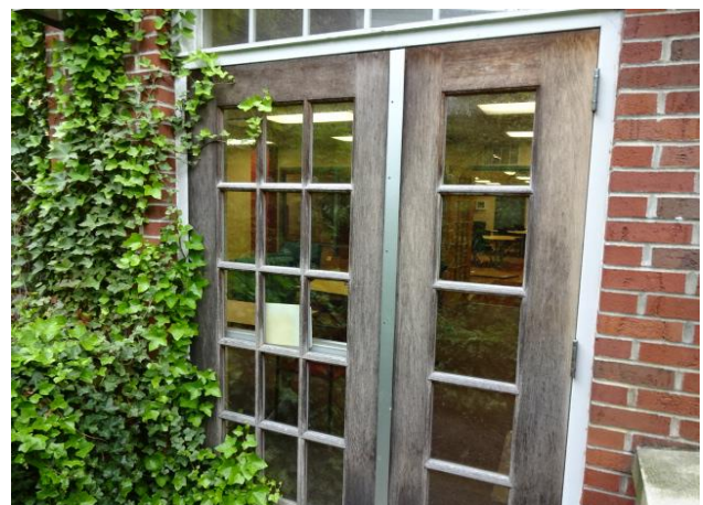
Wood Doors at Basement Level
