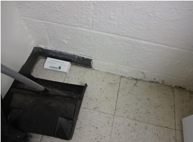
CMU Foundation Wall Interior
