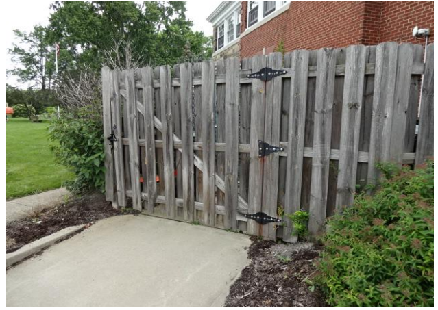
Dumpster Enclosure Fence
