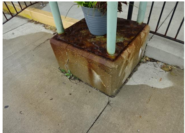
Entrance Canopy Foundation
