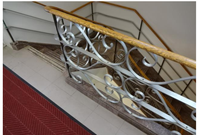
Handrail to be Replaced
