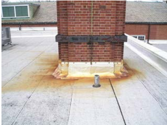
Steel straps are corroding and stack stability could be compromised.
