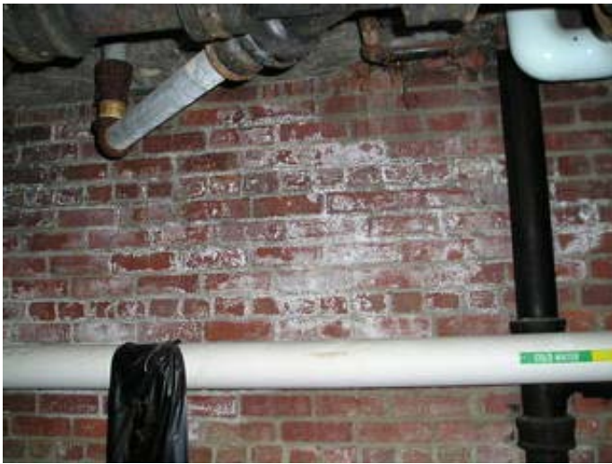
Efflorescence was observed on this tunnel wall
