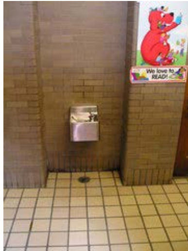
Drinking fountain not wheelchair accessible
