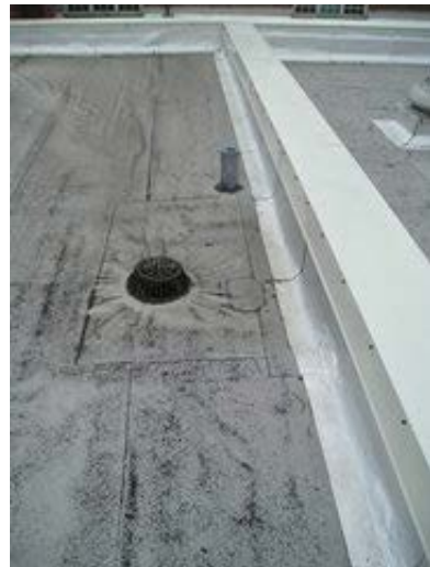
Evidence of ponding taking place several feet from point of drainage. Worn away top ply granules are collecting around this roof drain.
