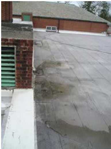
Evidence of ponding taking place several feet from point of drainage. Worn away top ply granules are collecting around this roof drain.
