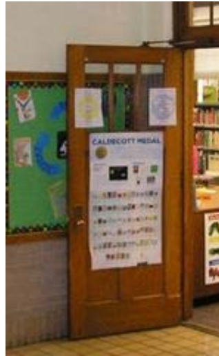
Door hardware is not ADA compliant
