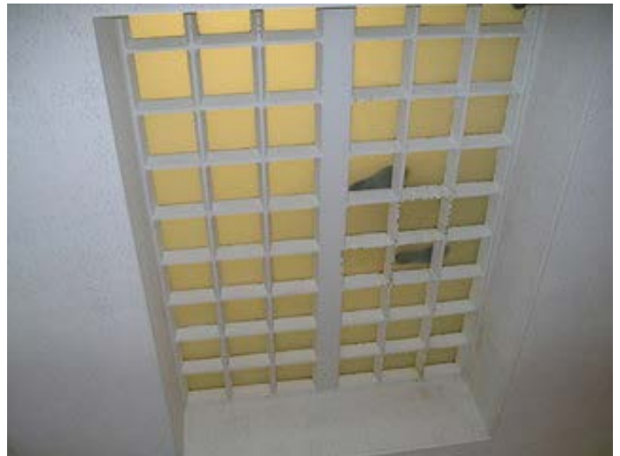
Glass block block in the floor may foster vertical fire spread
