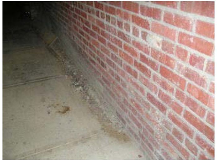
Moisture was observed on the floor near this tunnel wall
