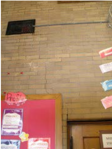
A crack leads from the upper left corner of this door
