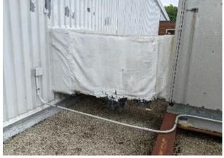
**Deteriorating Duct Insulation at Munters Unit**
