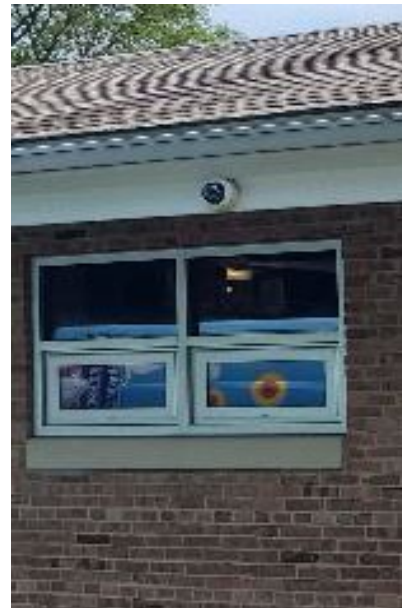
Exterior Security Camera
