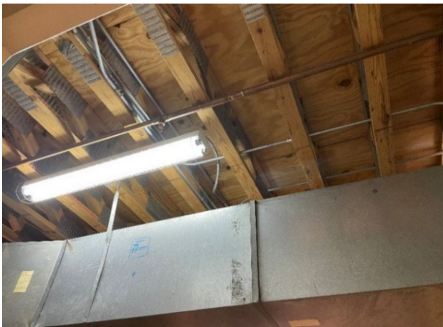
Wood Truss Joist Structure over Basement
