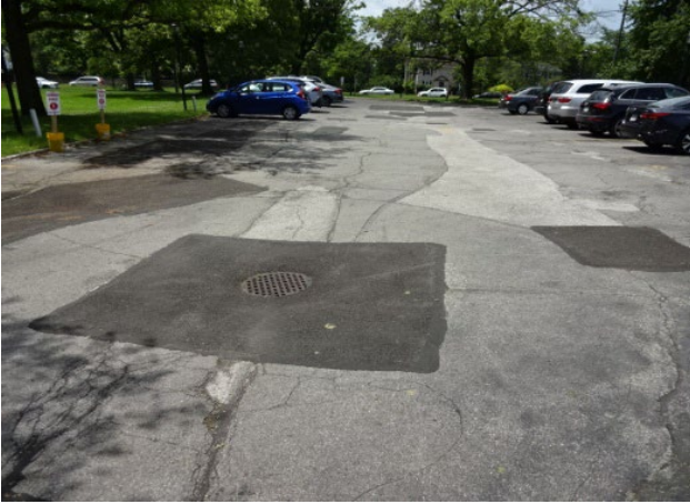
Asphalt Parking Lot
