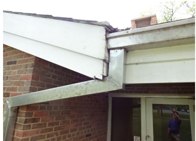
Wood Trim and Fascia
