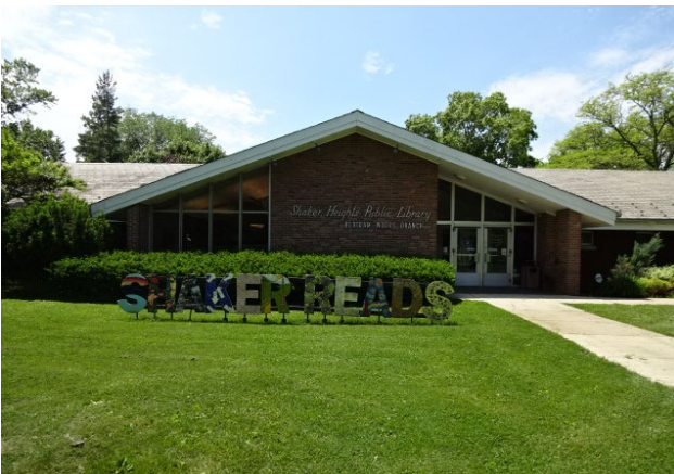
Main Entrance - Northeast Elevation
