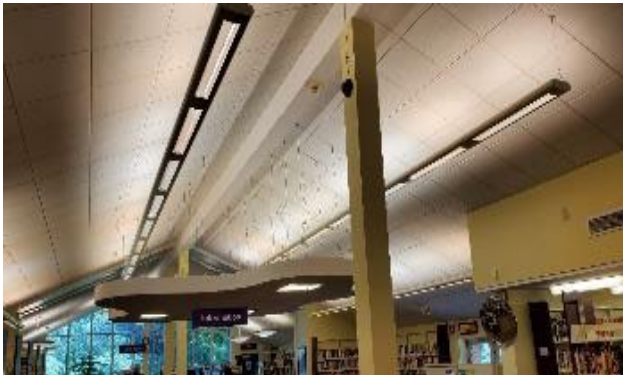
Linear Suspended T8 Fixtures
