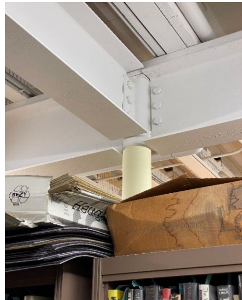
Steel Support Structure
