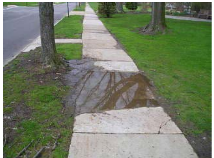
Standing water is present over this area of concrete walk.
