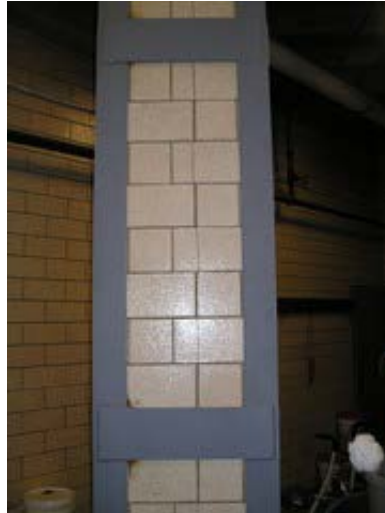
Vertical cracks were observed in this foundation pier.
