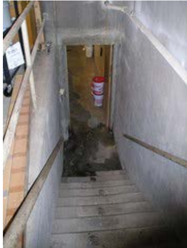
Water is breaching the foundation at the lowest levels.
