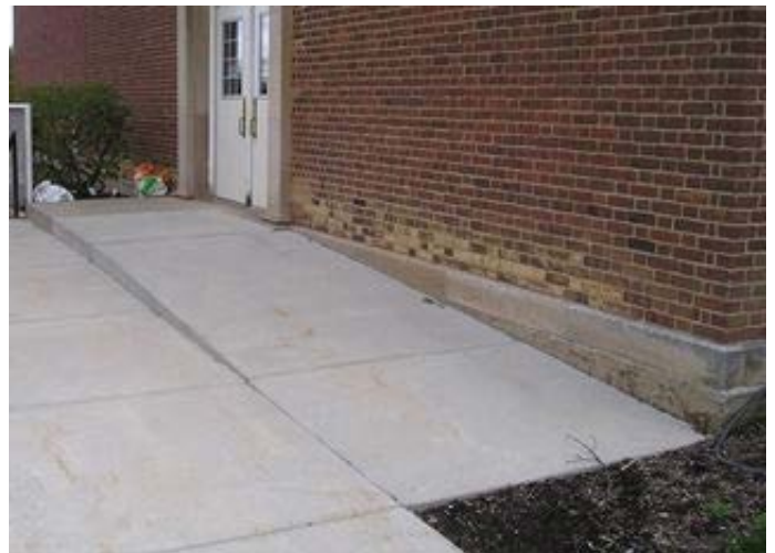
Surface damage to the face of this brick
