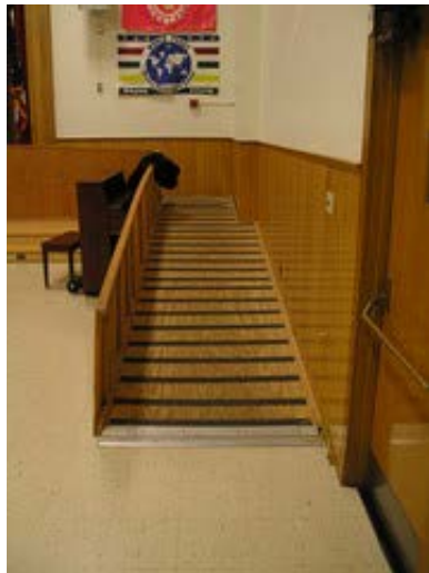
This ramp is steeper than 1:12
