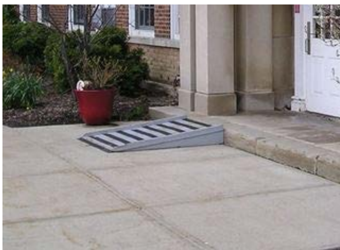
This temporary ramp should be replaced with concrete and rails
