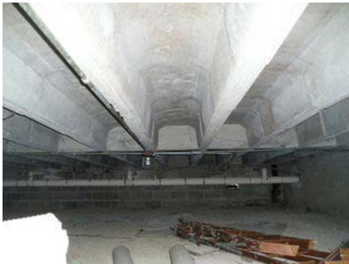
Concrete pan joists observed from crawl space
