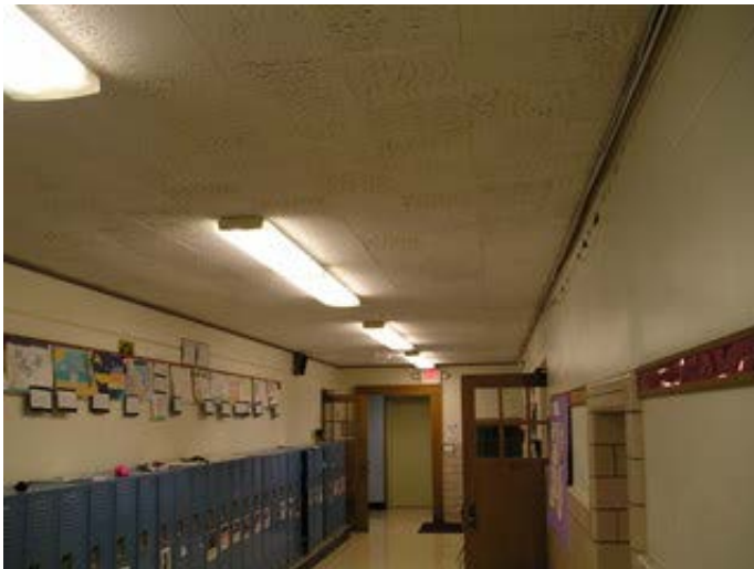
Finishes in a typical corridor
