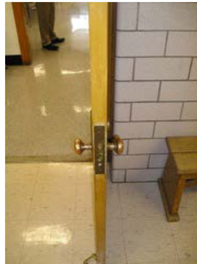
Door hardware is not ADA compliant
