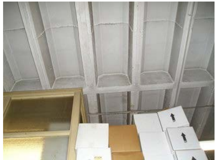
Concrete pan joists observed from mechanical room
