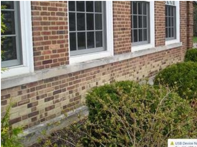
Surface damage to the face of this brick.
