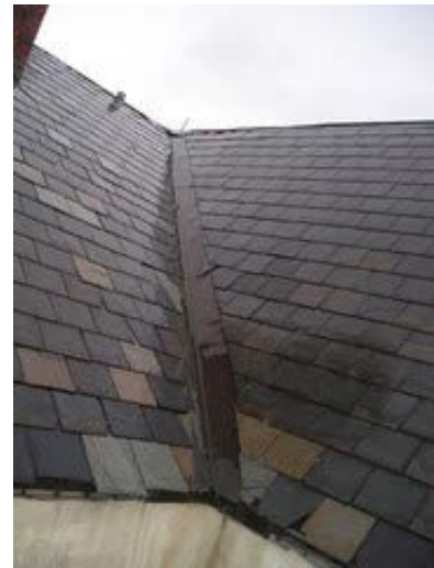
Damaged and replaced slate near valley
