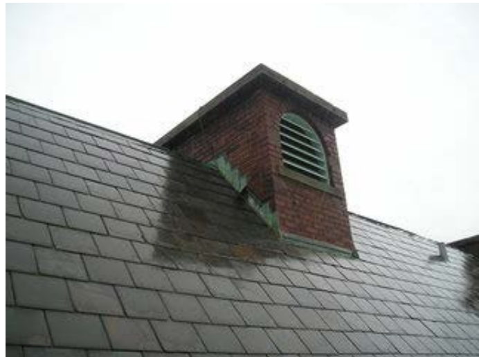
Flashing is damaged at this dormer
