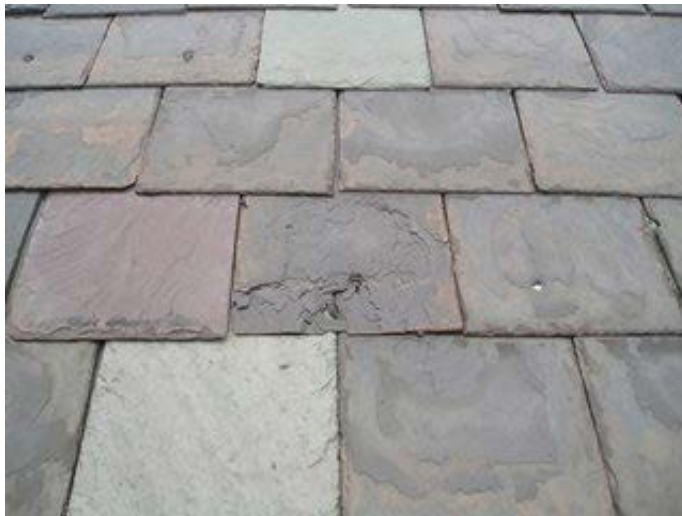
Damaged and replaced slate tile
