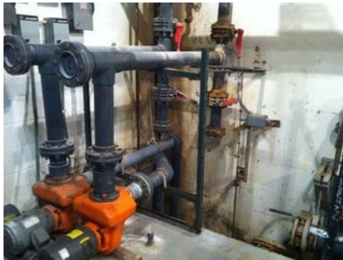
Storm water sump pump
