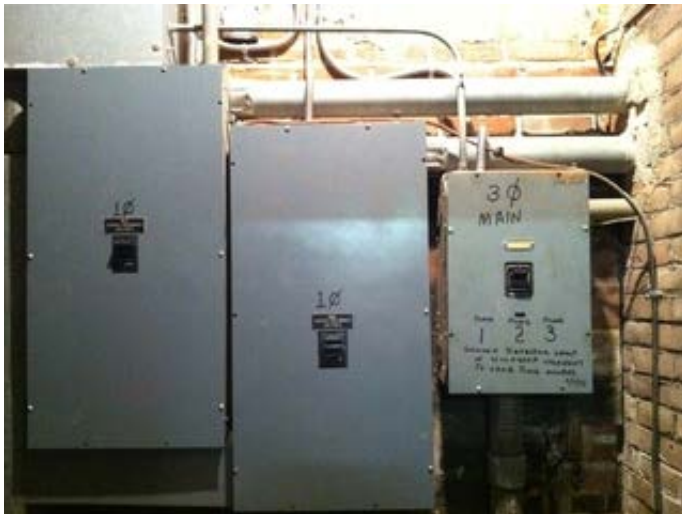
Main Electrical Switch Gear
