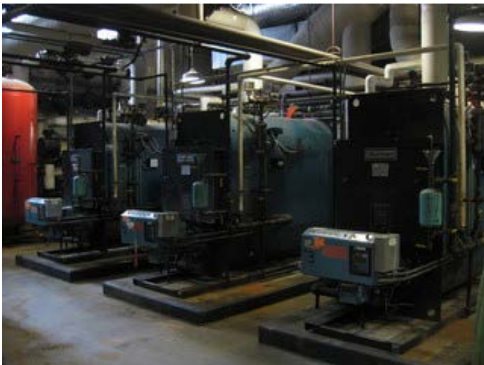
Main Mechanical Rm Steam boilers
