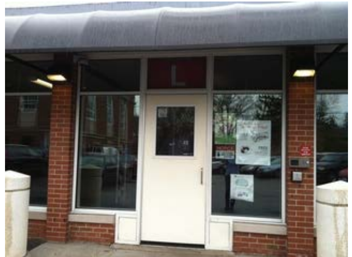
Front Entrance door
