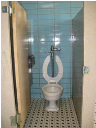
Floor mounted toilet
