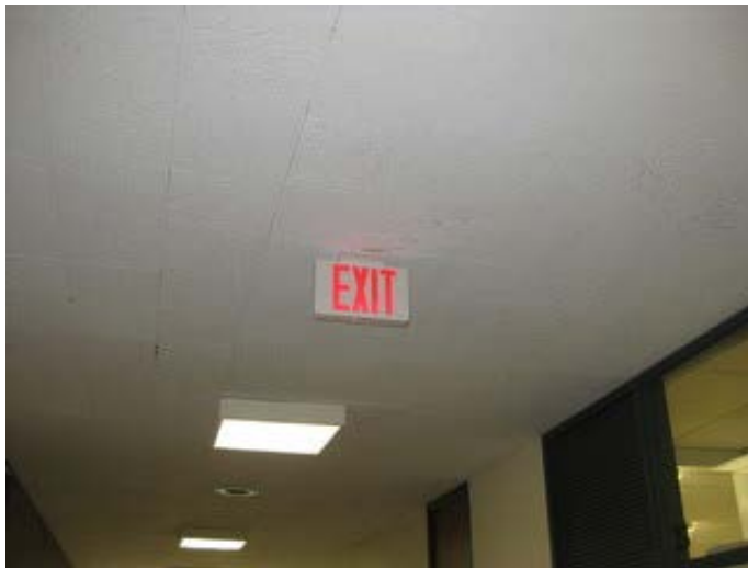
Emergency exit light
