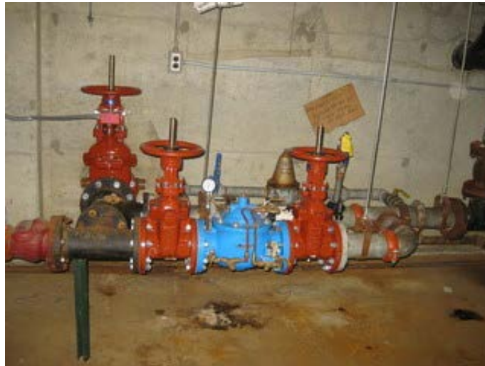
Pressure regulator at water entrance
