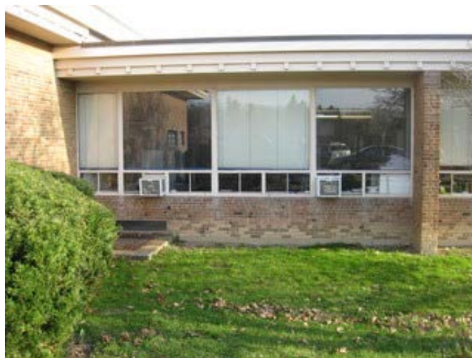
Window air conditioners
