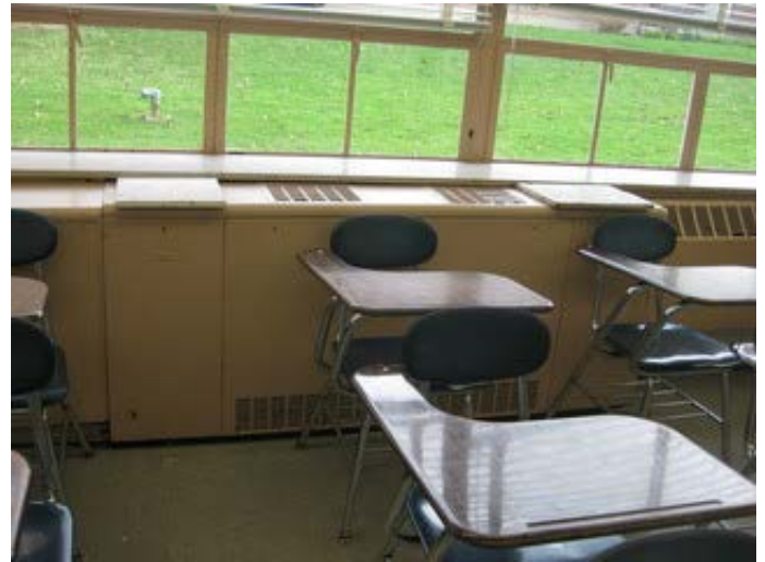
Classroom Unit Ventilator
