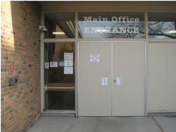
Security at Front Entrance Door
