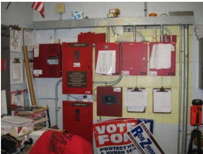
Main Fire Alarm panels
