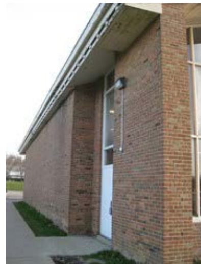
Exterior lighting near entrance
