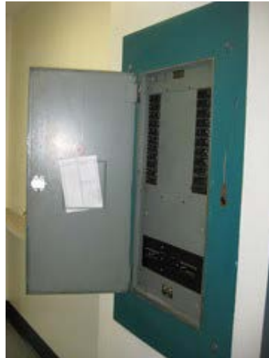
Panel Board mounted in corridor wall
