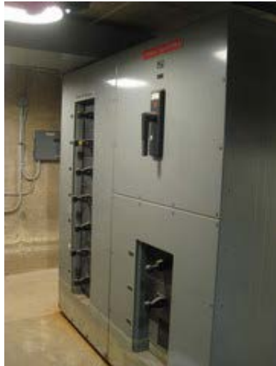
Main Electrical Switch Gear
