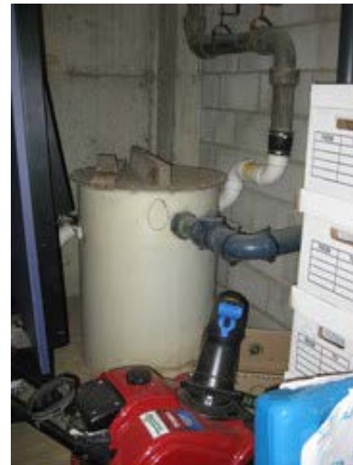
Acid neutralization sump
