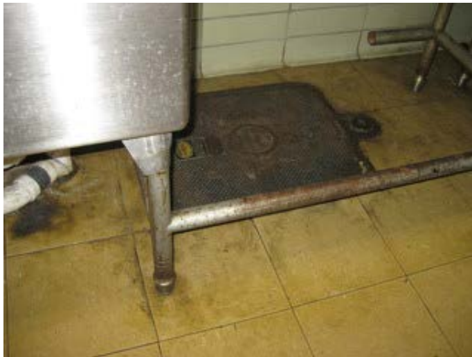
Kitchen Grease trap access
