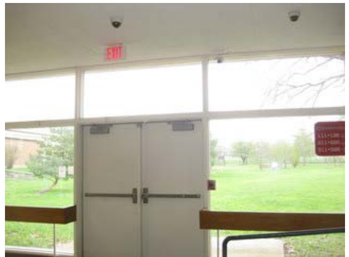
Fire Alarm devices
